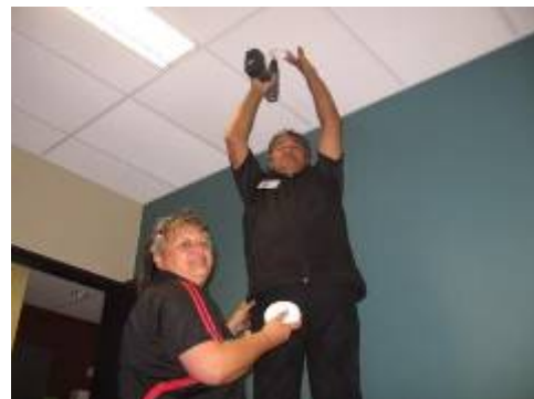
Installation of Smoke Alarms
