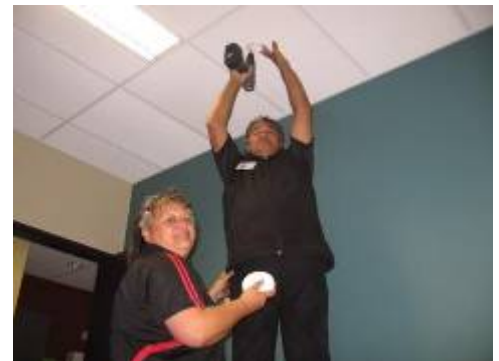
Installation of Smoke Alarms
