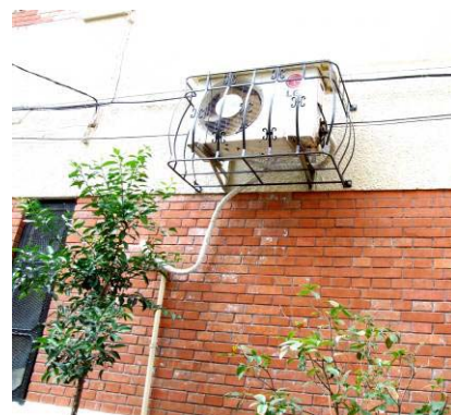
Renovated air-conditioning exterior equipment
