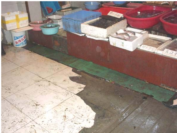
Food markets before renovation
