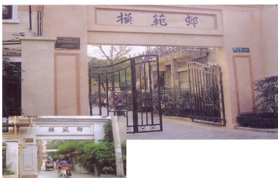
Residential quarter before and after renovation
