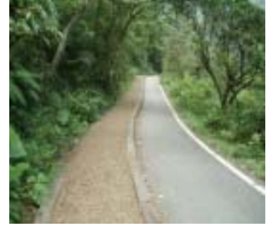
Fig. 37 To spread wooden materials for anti-slip
