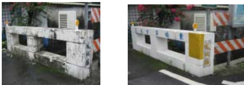
Fig. 29 Improvement for high-risk road, before(left) and after(right)
