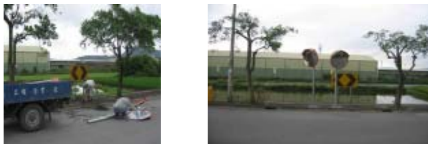
Fig. 30 Installation of reflection mirrors, before(left) and after(right)
