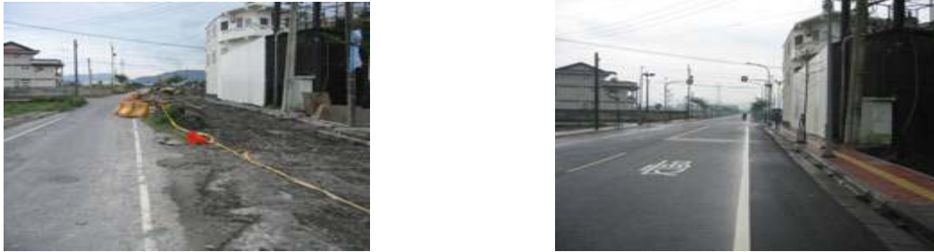
Fig. 28 Improvement for high-risk road, before(left) and after(right)
