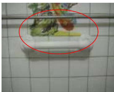
Fig. 16 After improvement, a suitable handrail in bathroom
