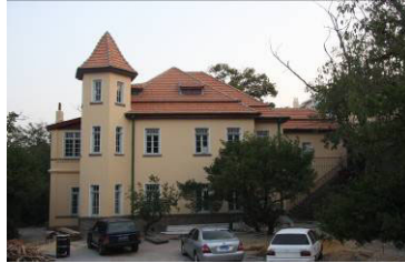
Rebuilt Damaged Building
