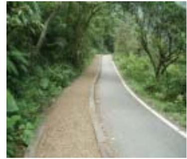
Fig. 37 To spread wooden materials for anti-slip
