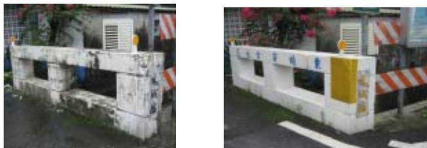
Fig. 29 Improvement for high-risk road, before(left) and after(right)
